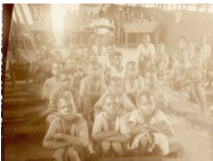
Classroom front view
