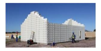
Housing and construction systems developer Moladi says its low-cost housing system, comprising plastic formwork panels and a cement admixture, is widely embraced throughout Africa, as it has been specifically designed to meet the requirements of the African market.
