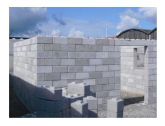
These blocks can be made in the same size as standard concrete blocks, though don't have the same weight-bearing capabilities. The blocks do have good acoustic and thermal insulation properties, which ByFusion says makes them ideal for use in road projects or fill-in building frames.
