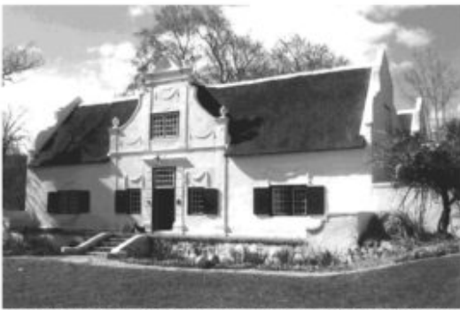
Figure 10.1 The real thing. The homestead of Nieuwe between Somerset West and Stellenbosch, built in 1814. The real 'place of memory': the face of the house is its gable, not the thatch roof, the casement windows and the H-plan, which are standardized. (Photo: author)
