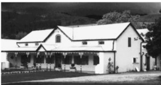
Figure 10.2 To hell with all these places of memory! Here the loss of the gables is somewhat compensated by the Victorian veranda with imported cast-iron work. Nabygelegen is situated in the Bovlei, near Wellington, not far from where the Afrikaans 'language movements' took place at around the same time. (Photo: author)
