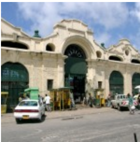
Mombassa Market Hall
