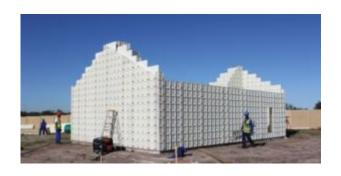
Housing and construction systems developer Moladi says its low-cost housing system, comprising plastic formwork panels and a cement admixture, is widely embraced throughout Africa, as it has been specifically designed to meet the requirements of the African market.
