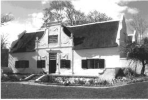
Figure 10.1 The real thing. The homestead of Navarre between Somerset West and Stellenbosch, built in 1814. The real 'place of memory': the face of the house is its gable, not the thatch roof, the casement windows and the H-plan, which are standardized. (Photo: author)
