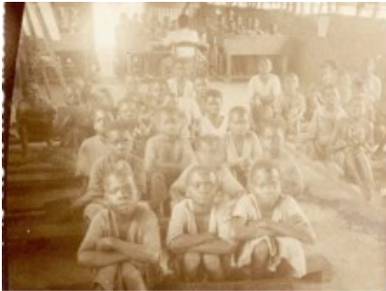
Classroom front view
